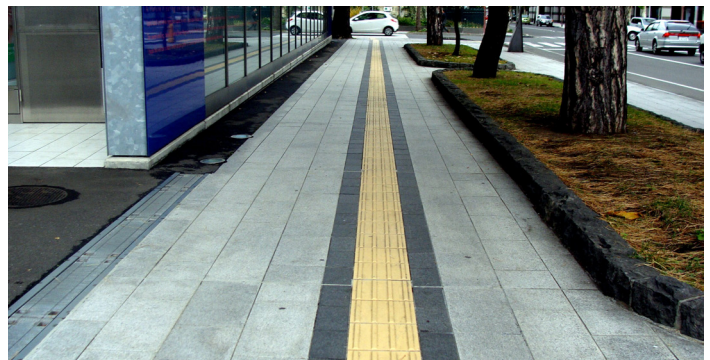
Tactile Paving Used to Guide the Visually Impaired. Source: Streets of Louga
